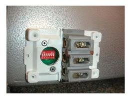
Settings are adjustable via DIP switches located inside Generator Input Junction Box.
